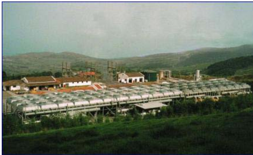
Figure 3 – Sao Miguel Geothermal Power Plant
