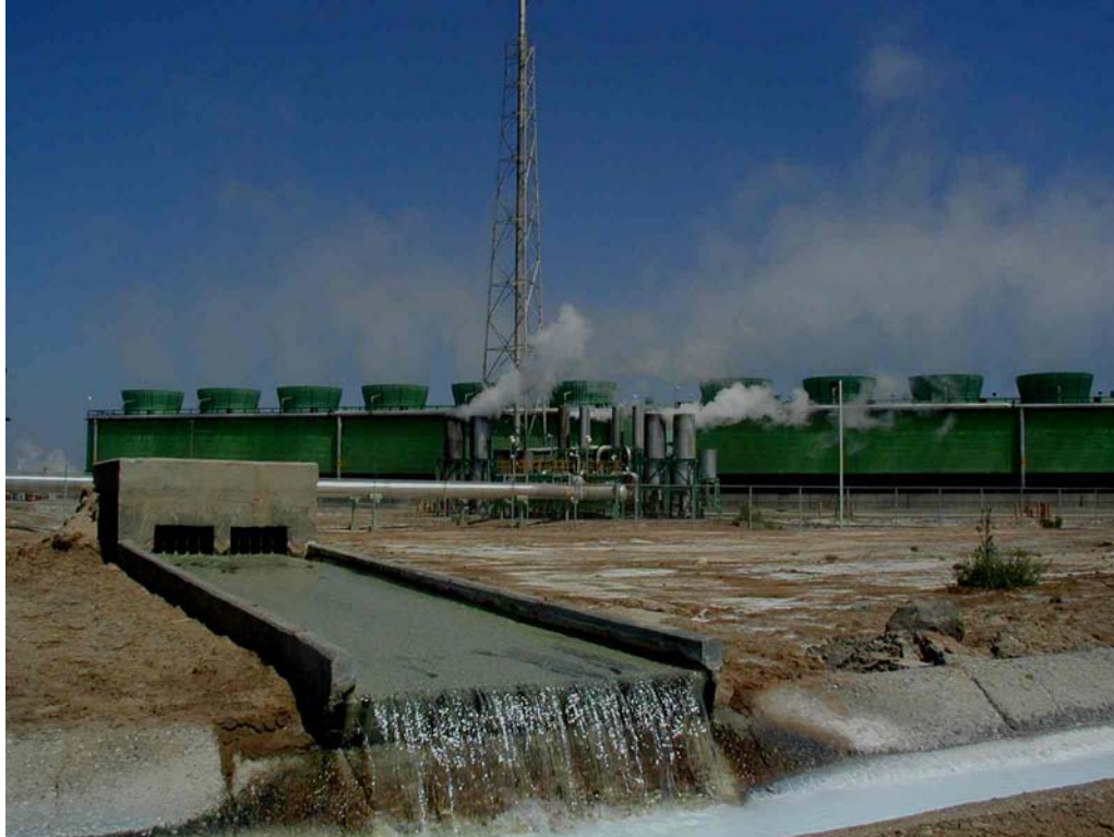
Figure 1. Cerro Prieto IV 4x25MW Facility, Owned by Comisión Federal de Electricidad, of México.
