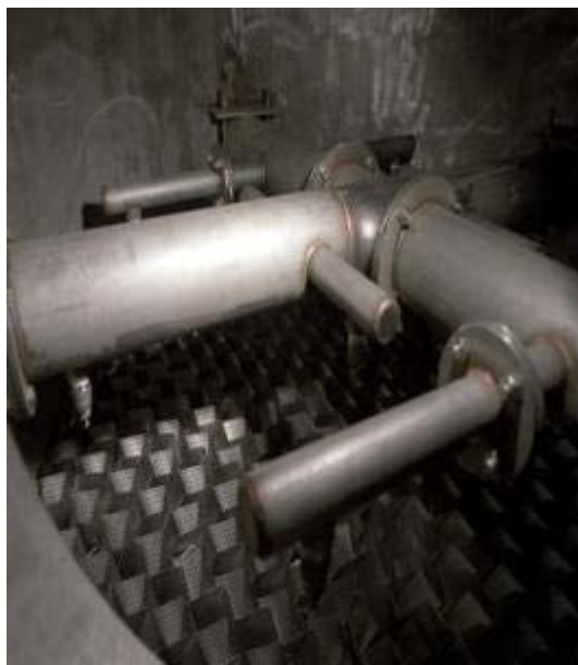
Figure 4. Headers that Distribute Condensing Water onto the Packing.
