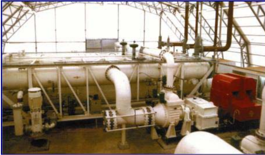
Figure 6 – Svartsengi Exhaust Steam Recovery Project, Iceland
