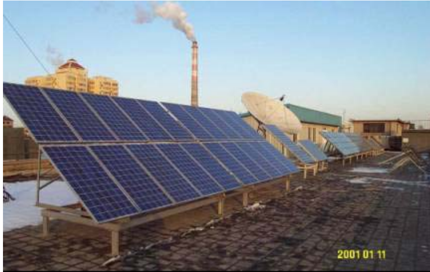
Figure 11: ATS 10 KW Solar Photovoltaic System
