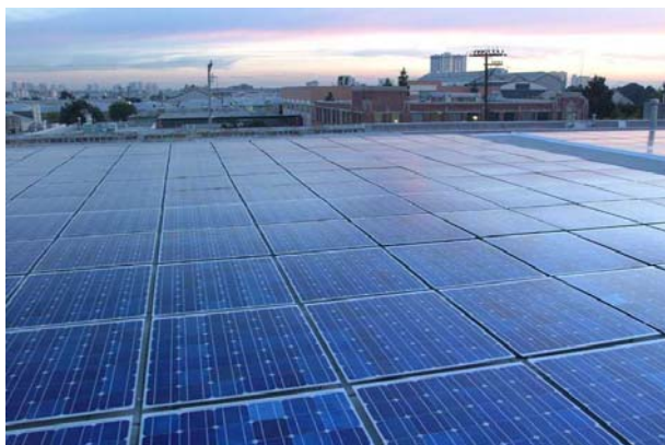
Fig. 5. This 100-kilowatt Berkeley, CA power plant is composed of 39,000 state-of-the-art AstroPower solar cells.
