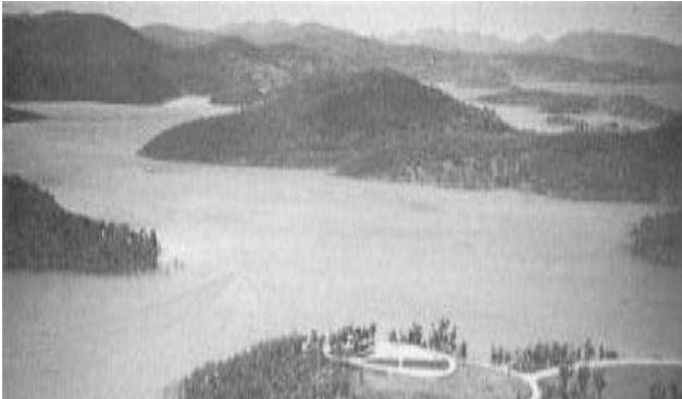
Fig. 2. Eucumbene Dam in the Snowy Mountains in Australia
