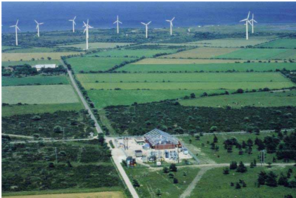
Figure 5. The Gotland VSC HVDC project in the foreground. Wind power in the background
