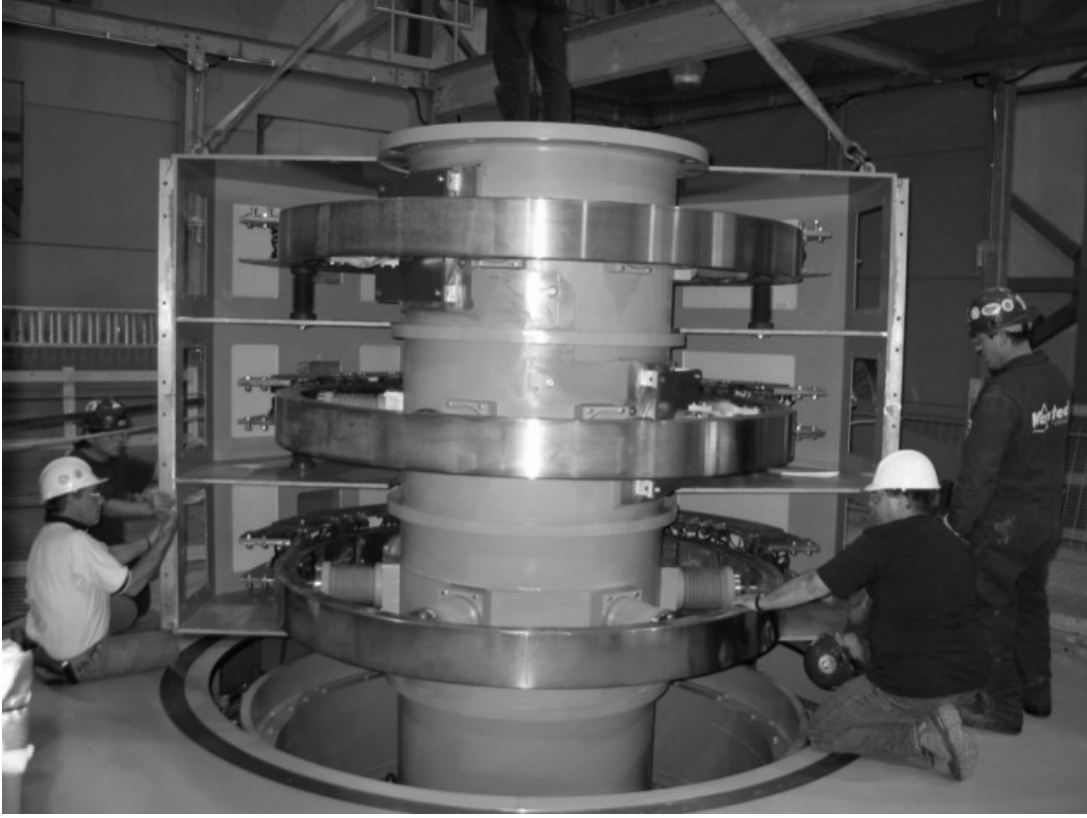
Fig. 5. A typical assembly of VFT three phase collector.
