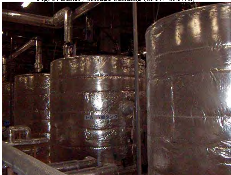
Fig. 4. Battery storage tanks
