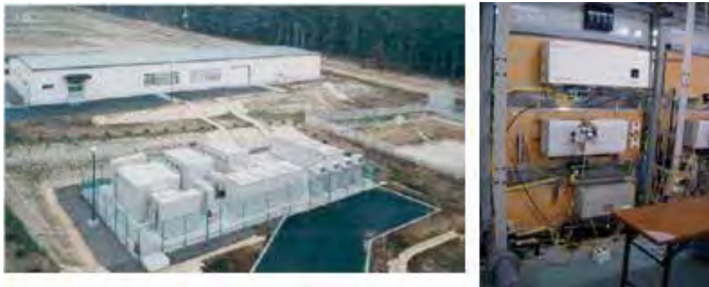
Fig. 13. Islanding prevention test facility in Maebashi
