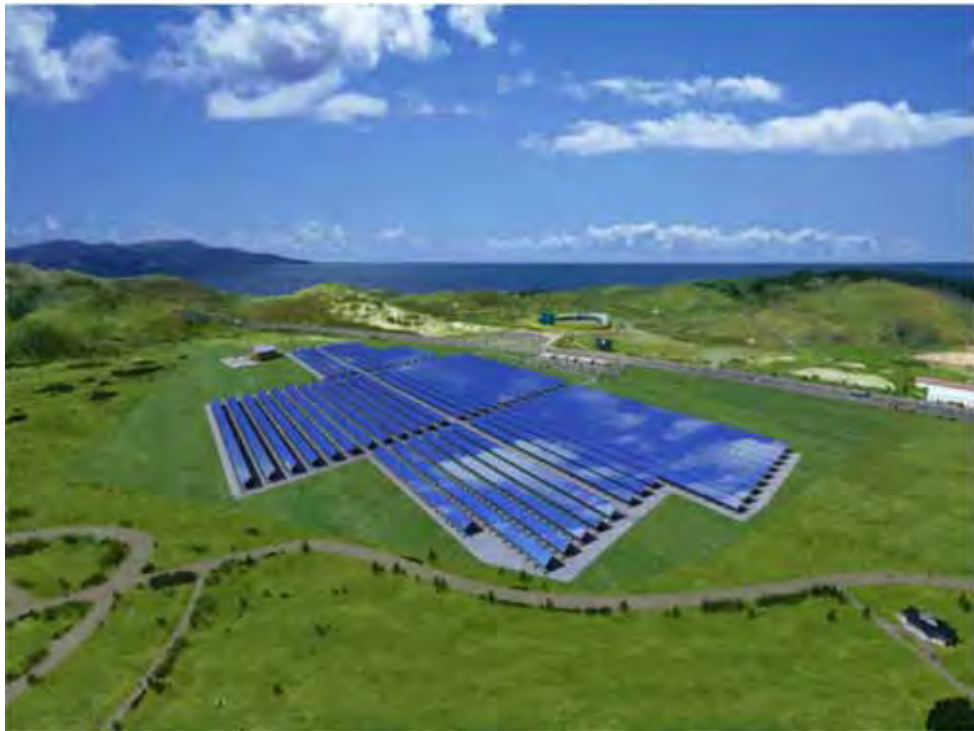
Fig. 6. Image of Wakkanai PV power generation system
