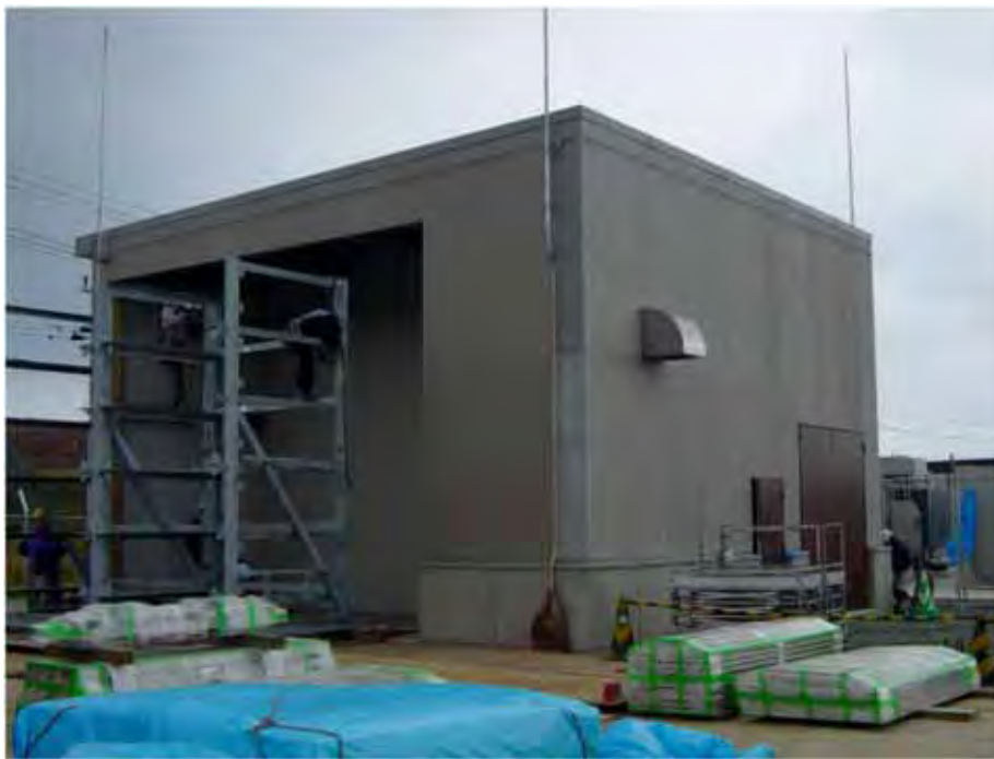
Fig. 8. Construction of battery storage building (500kW-3.5MWh)
