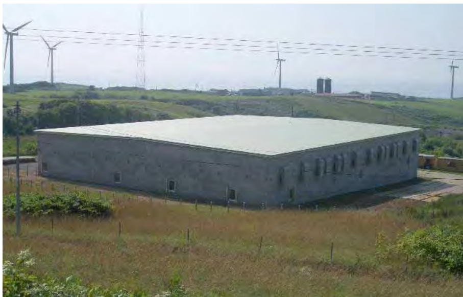
Fig. 3. Battery storage building (6MW-6MWh)
