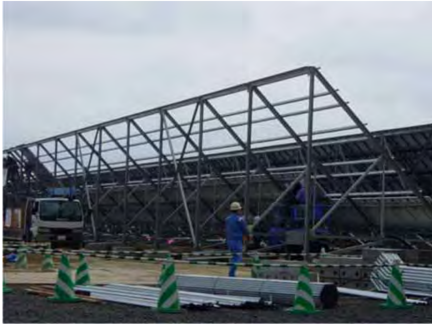
Fig. 9. Installation of PV panels in Wakkanai
