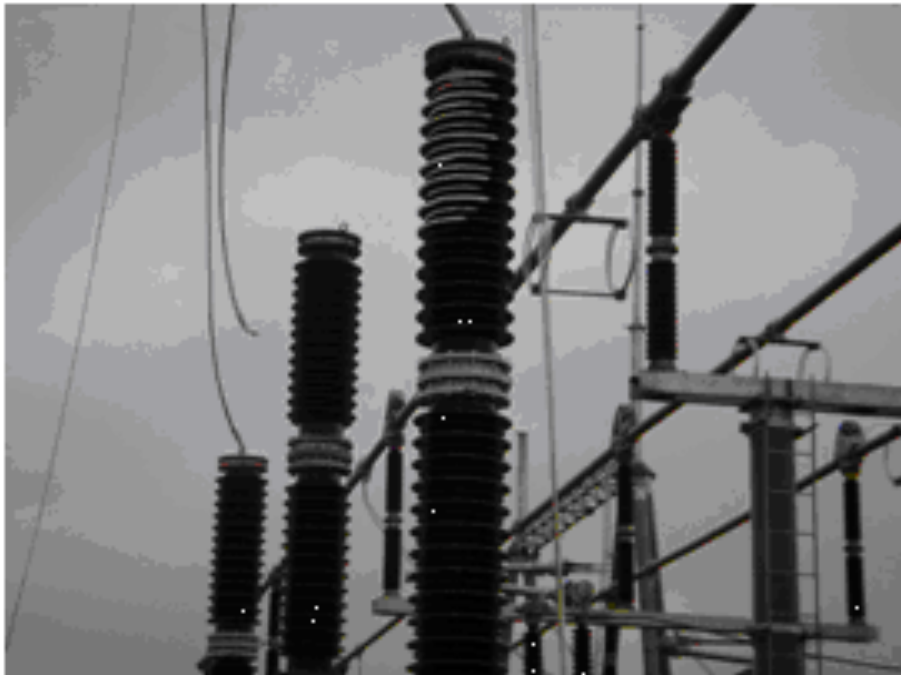
Fig.2 The short fault on b phase to c phase of the coupling capacitor.
