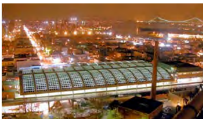
Fig. 2. Coney Island Subway Terminal of New York City Transit Authority - 300 kW (2X150)
