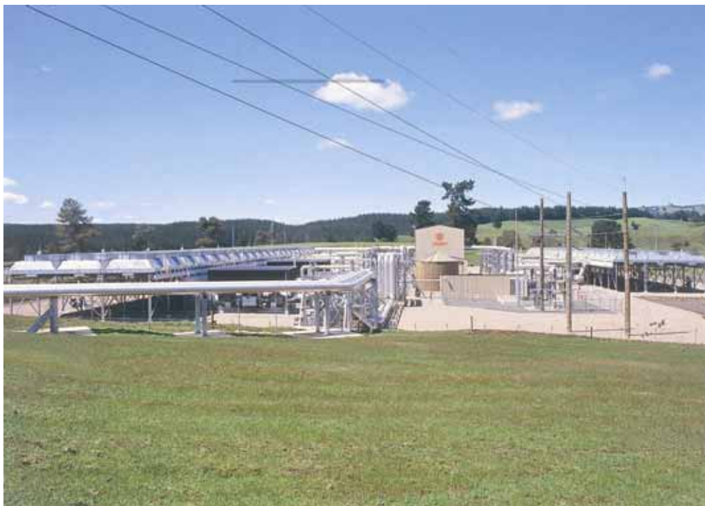
Fig. 17. 100 MW Mokai 1 and 2 Geothermal Power Plants in New Zealand
