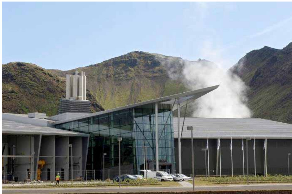
Fig. 4. Hellisheiði power plant.
