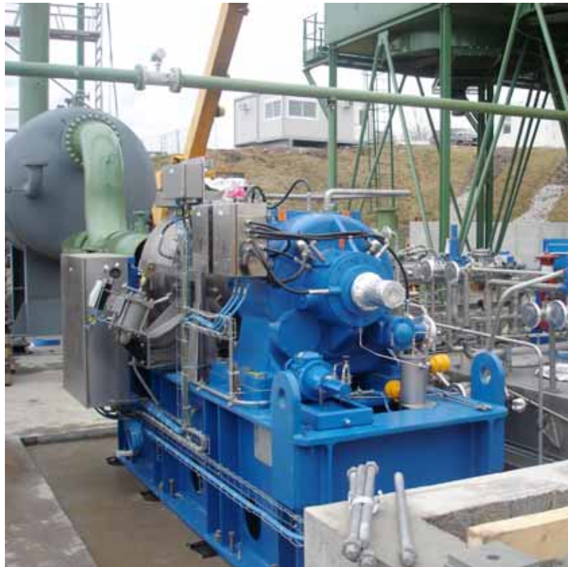
Fig. 12. The turbine being installed.
