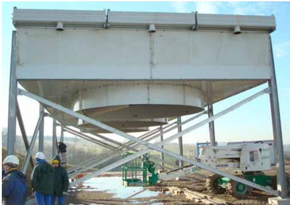
Fig. 14. The second air-cooling system being installed.
