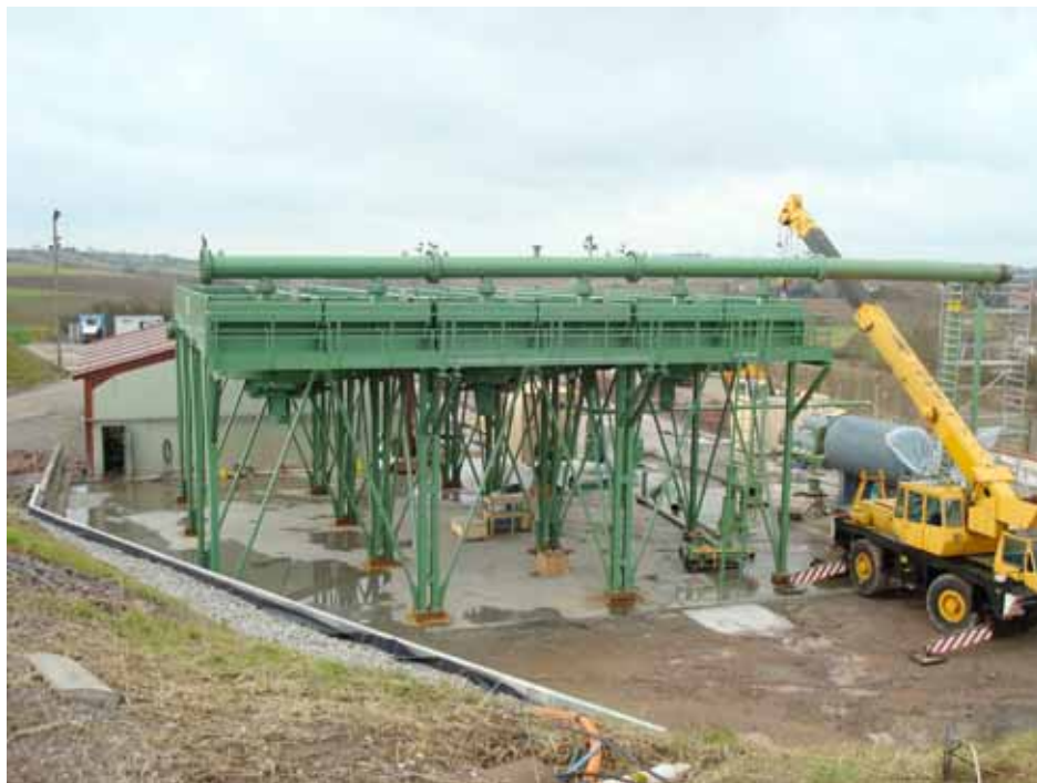
Fig. 11. Installation of the air-cooling system
