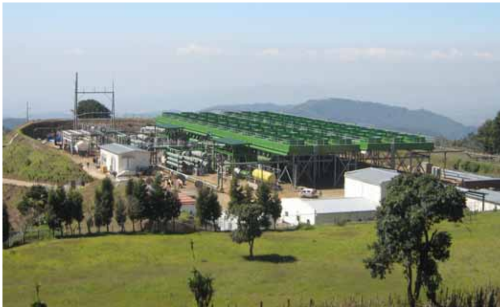
Fig. 13. 20 MW Amatitlán Power Plant in Guatemala
