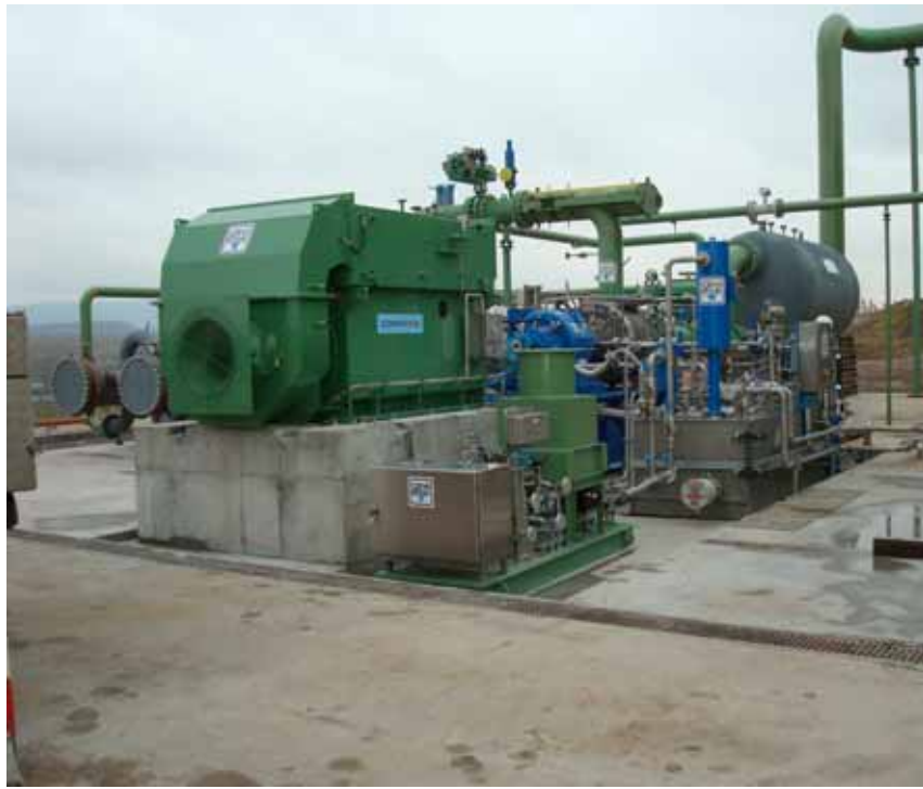
Fig. 13. Generator (foreground) aligned with the turbine.
