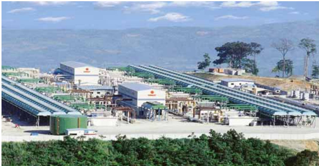
Fig. 16. 125 MW Upper Mahiao Geothermal Power Plant in the Philippines
