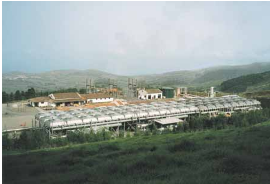
Fig. 5. Two-phase 14 MW Ribeira Grande Plant in the Azores
