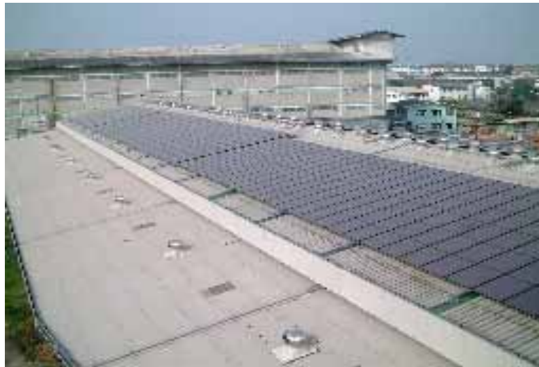
Fig. 2. PV arrays on rooftop of warehouse
