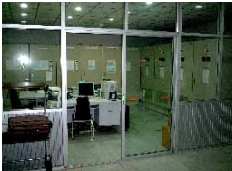
Fig. 3. Inside of Control Room
