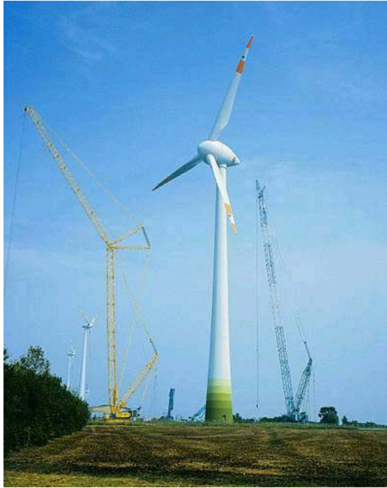
Figure 4. The ENERCON E112, a 114 metre diameter wind Turbine, hub height 124 metre, with a direct drive variable speed generator rated at 4.5 MW.
