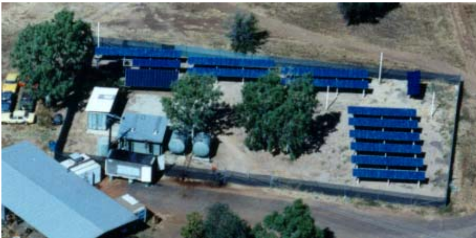
Figure 2. Photovoltaic array as part of a Hybrid Remote Area Power Supply at Jilkminggan in the Northern Territory of Australia. - Designed Constructed and Operated by the NT Power and Water Authority
