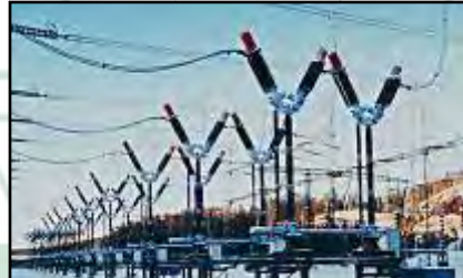
420 kV Oil minimum CB
