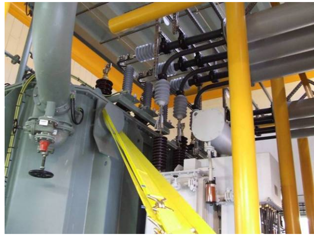
Fig. 9. 33 kV/132 kV transformer, 180 MVA
