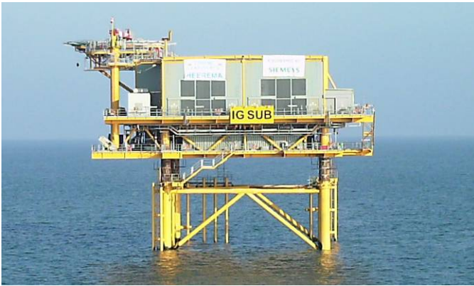
Fig. 8. Greater Gabbard Main Platform
