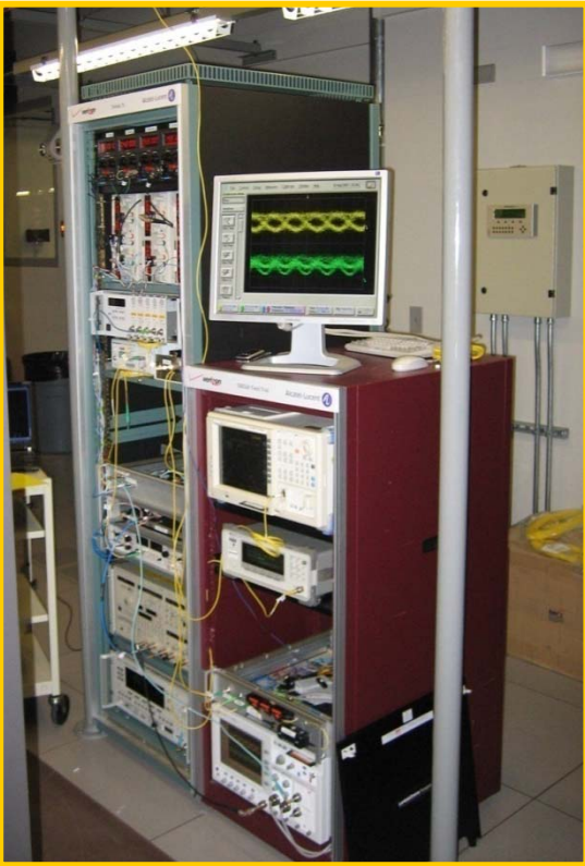
100G Transmitter at the Tampa Central Office
