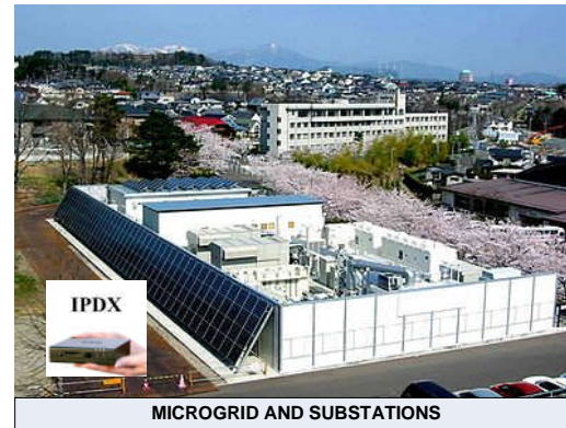
MICROGRID AND SUBSTATIONS
