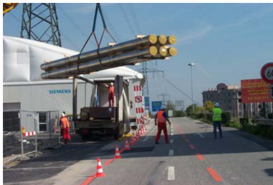
On site installation using a prefabrication tent
