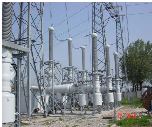
T&D Chicago MTS Mixed Technologies Switchgear
