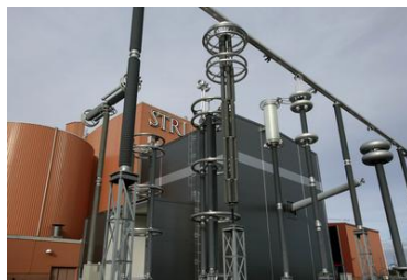
Long term test circuit for 800 kV HVDC
