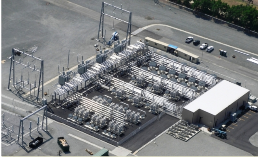
Dynamic Voltage Support with the Rector SVC in California's San Joaquin Valley FACTS PANEL SESSION, IEEE/PES T&D Conf. & Expo, Chicago, IL - April 23, 2008
