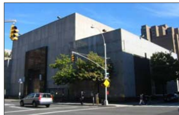
138kV-13kV Manhattan Area Substation
