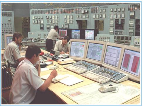
SPDS realized critical safety functions of monitoring in all NPP operation modes with the aim of identifying the signs of violation of critical safety functions and definition of personnel actions which are priority from safety point of view. These systems were designed by Westinghouse Electric Corporation (USA). "Westron" (Ukraine) provided development and implementation of these systems.
