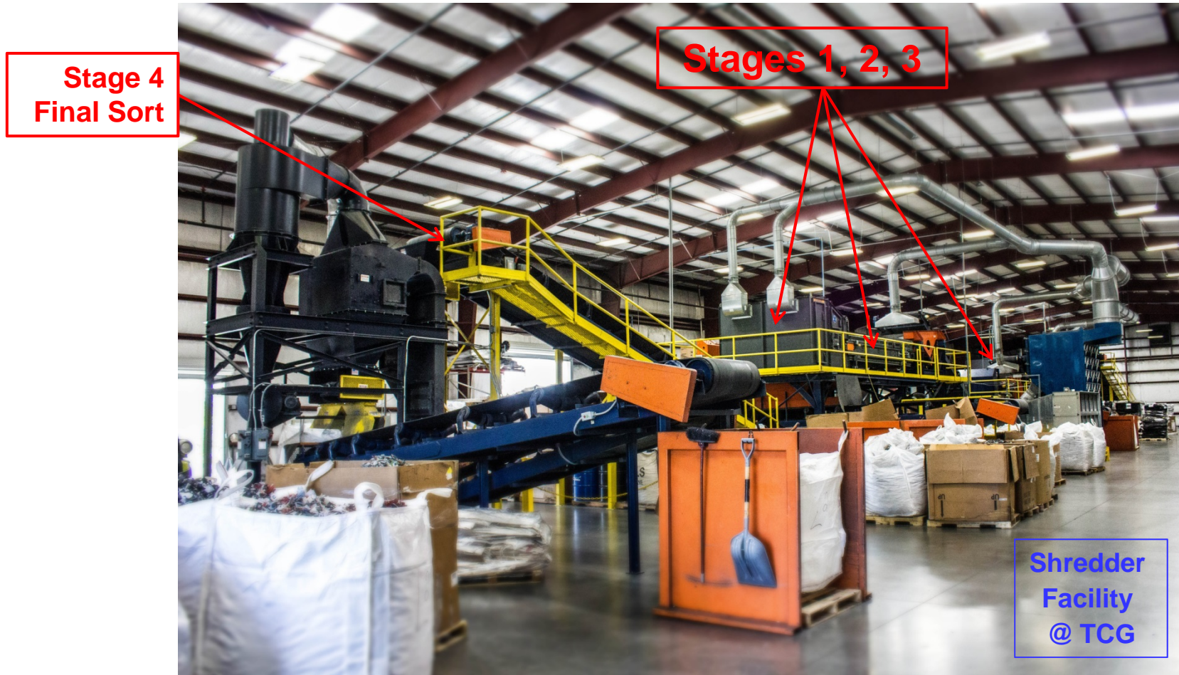
Automated Industrial shredder, Sorts & bins de-constructed materials
