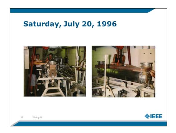
Here I am at NES removing their set of microwave cavities, or "waveguide" as they called it. All that can be seen is the smooth solenoidal magnet around the entire structure.
