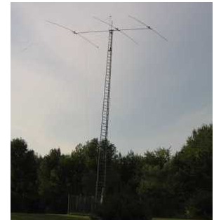
One of the Two 80' Towers
