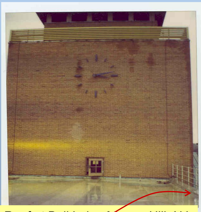
Roof at Bell Labs, Murray Hill, NJ. Card rack was here facing south.
