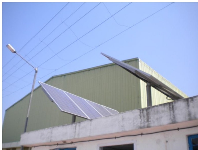
Fig: 2 Street Light applications of solar modules
