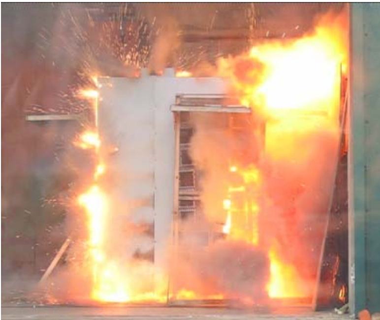
Fig #1 - 65kA Bus Compartment Arc
