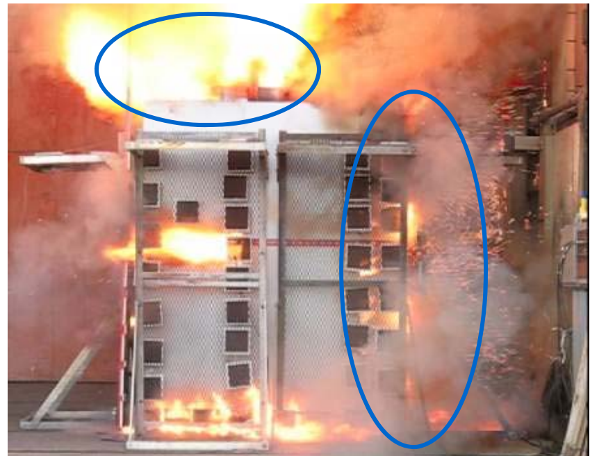
Fig #2 - 85kA Bus Compartment Arc
