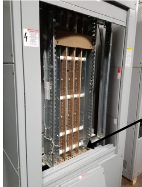
Low Voltage Switchboard
