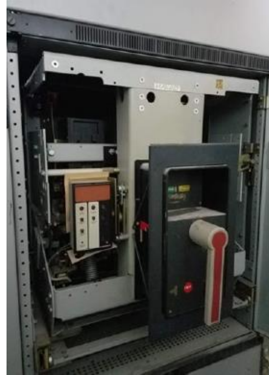
600V Drawout Switchgear with Iron Frame
