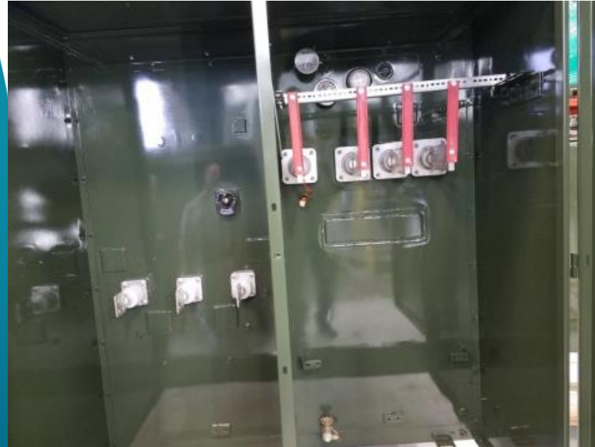
15kV / 480V Transformer compartments
