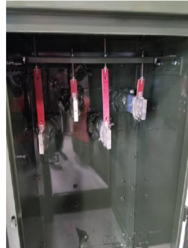
480V Transformer compartments
