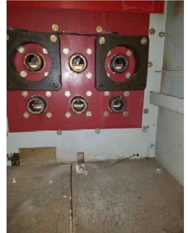
600V Drawout Switchgear breaker compartment
