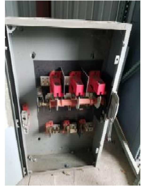
Low Voltage Fused Disconnect
