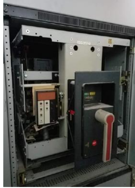
600V Drawout Switchgear with Iron Frame
