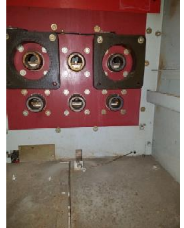
600V Drawout Switchgear breaker compartment
