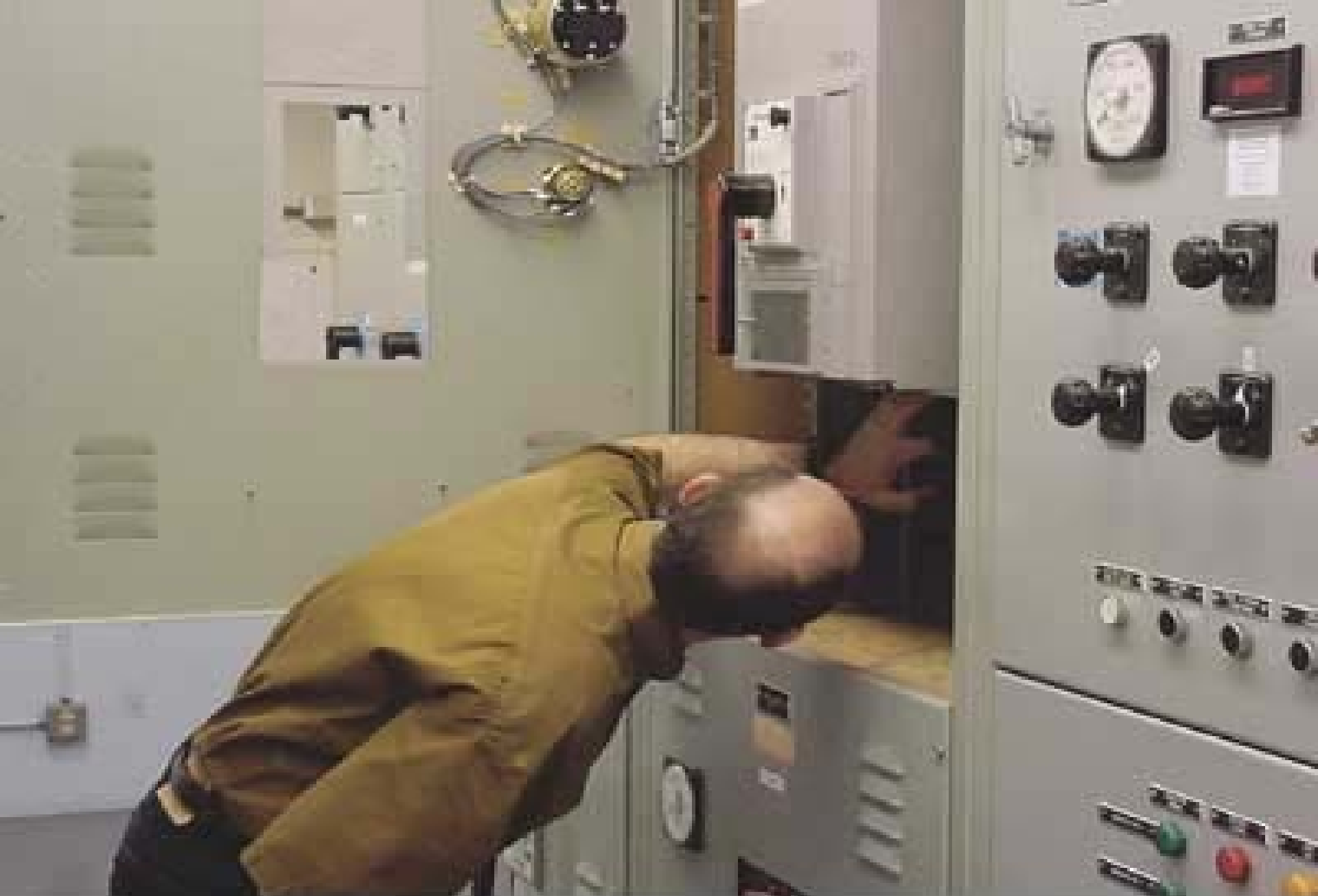
Photo 8. Inspector examining electrical equipment.
