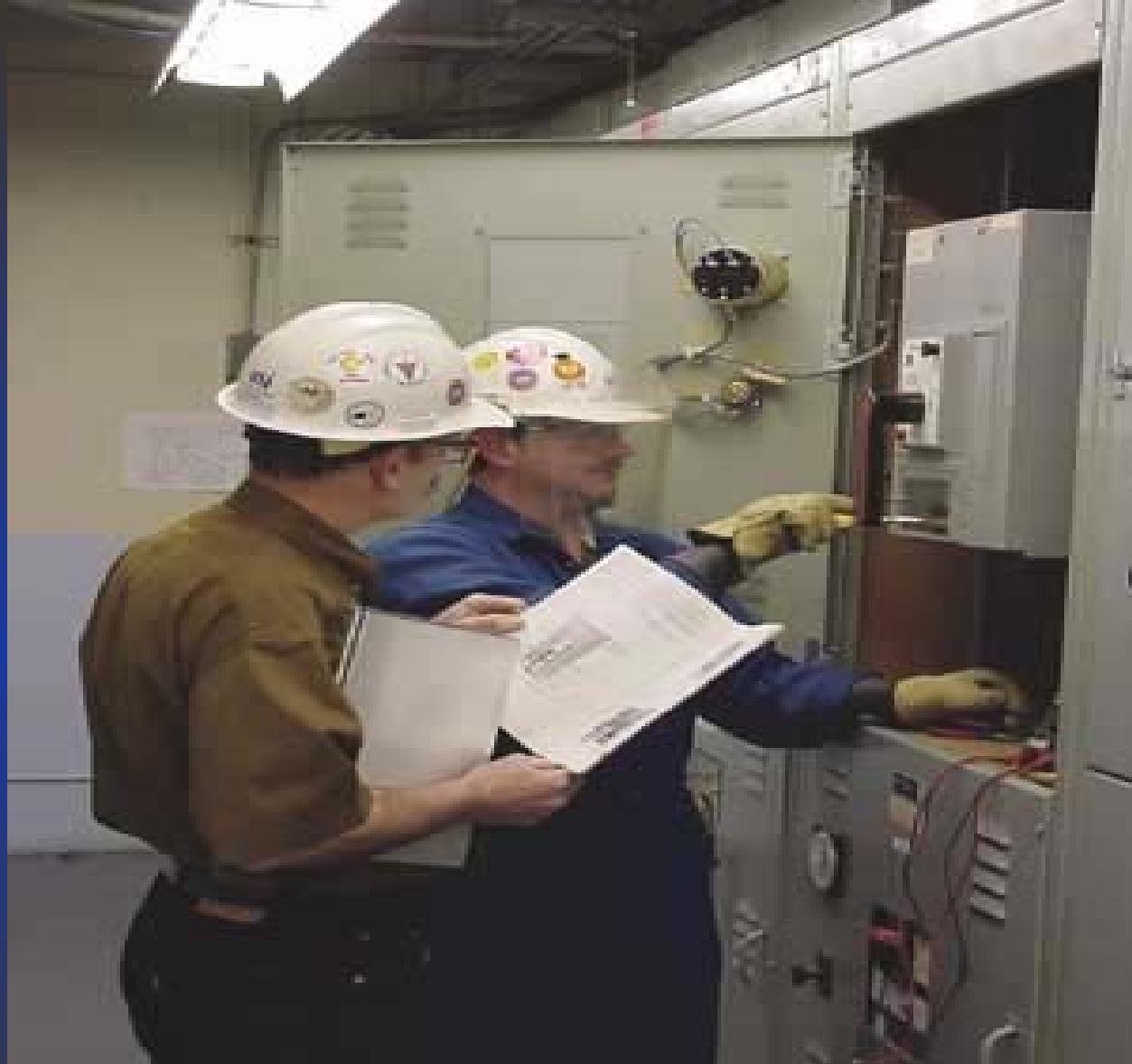
Photo 10. Workman is properly protected and inspector is shown in the flash hazard boundary in front of the switchboard with no personal protective equipment. If this equipment is energized, what is wrong with this picture?
