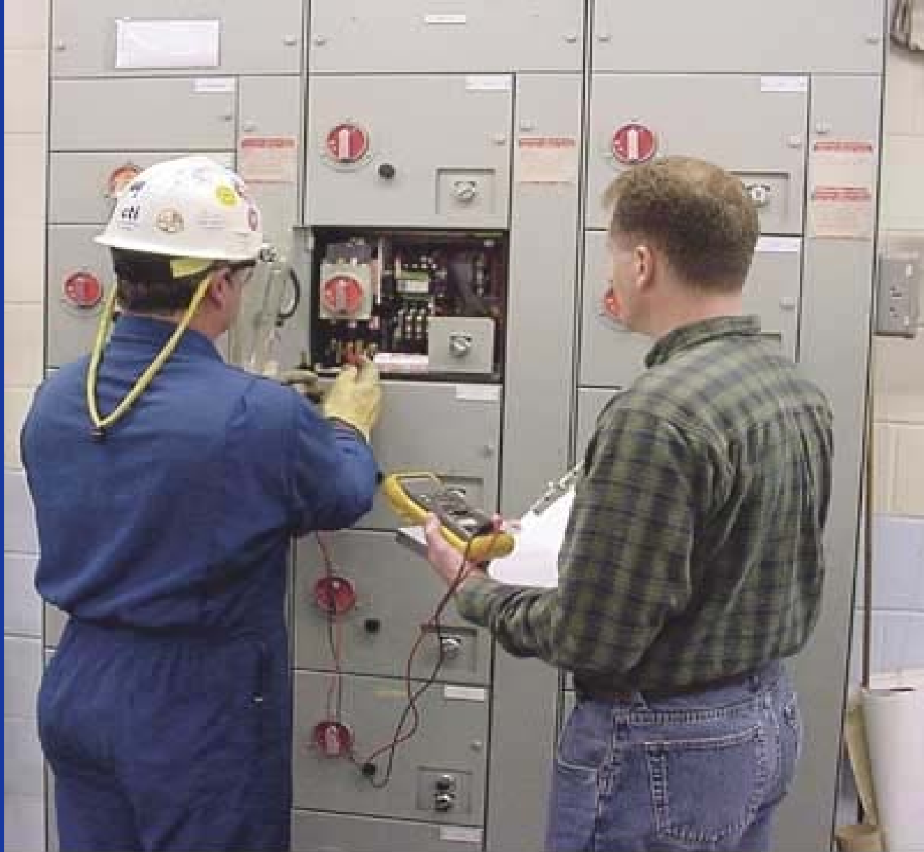
Photo 11. Workman is properly protected and inspector is shown in the flash hazard boundary in front of the motor control center. If this equipment is energized, what is wrong with this picture?
