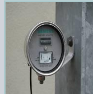
Arrester monitor with remote indication 3EX5 060/062
