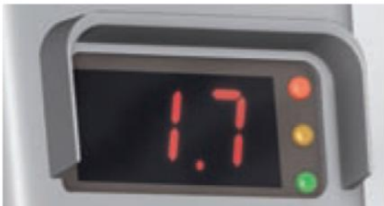
Display of leakage current
