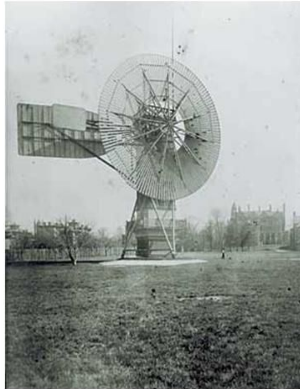
Charles Brush (1887-1888, Cleveland, Ohio) 1 st Automatically Operating Wind Turbine Generator 12kW, 17m Rotor Diameter Ran for 20 Years To Charge Batteries in Mansion Cellar www.windpower.org/en/pictures/brush.htm
