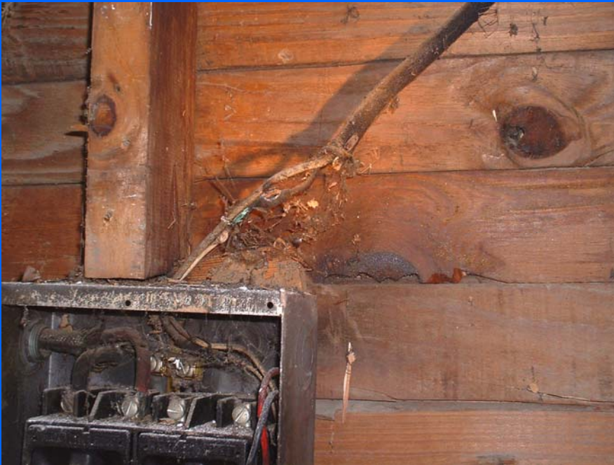
Improper Splice Glowing Red-Hot
