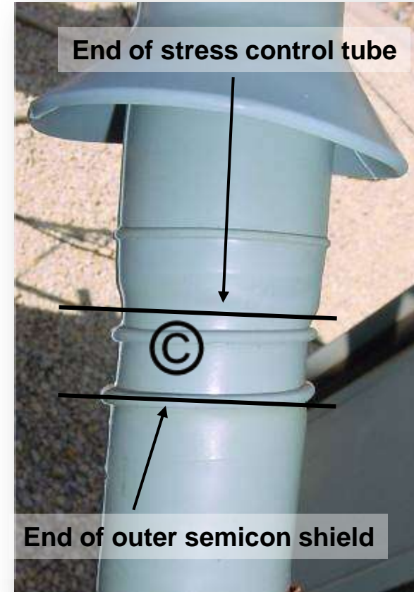
Example of misplaced stress material
