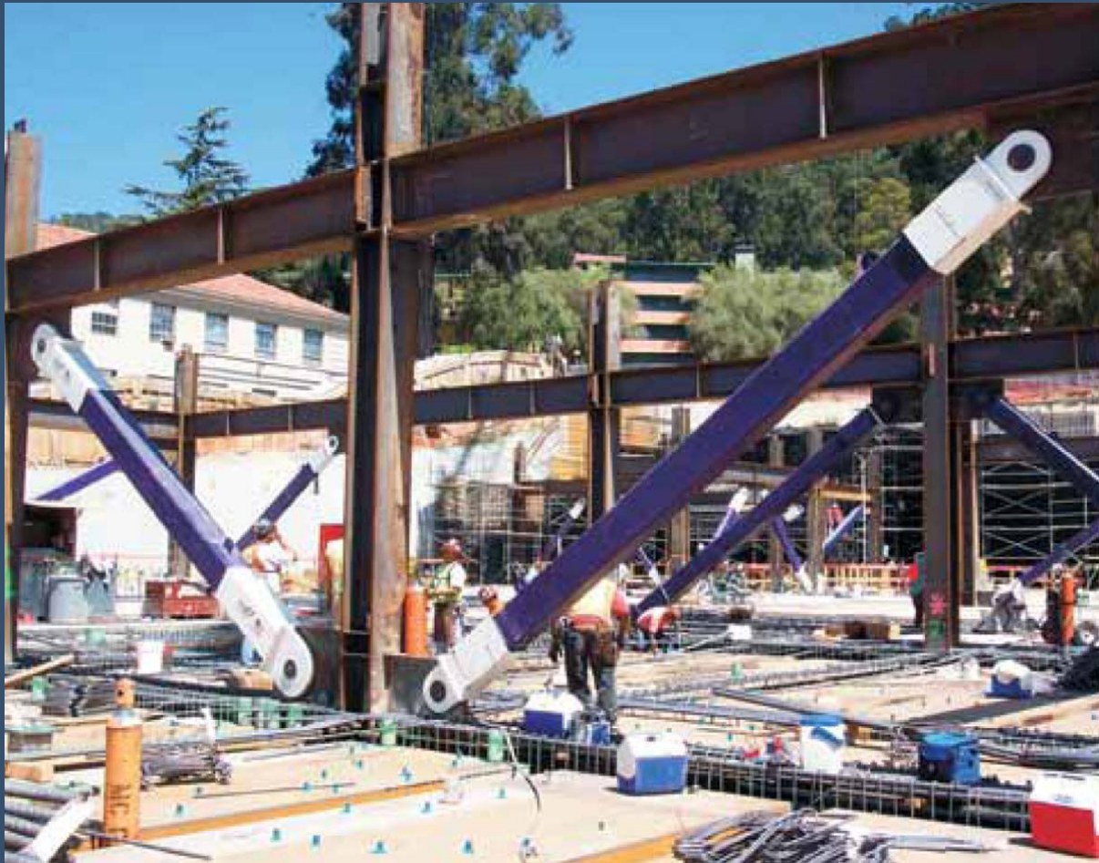
UC Berkeley Stanley Hall Replacement Project (2003)
