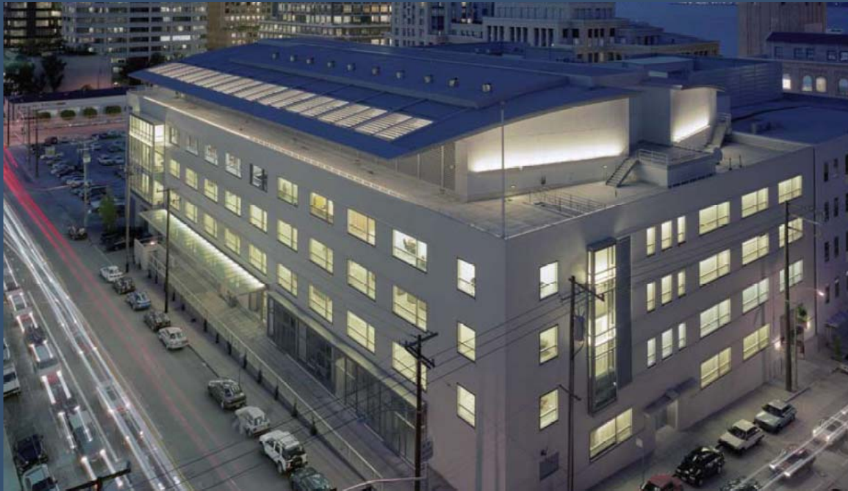
365 Main Data Center (2002) San Francisco, CA
