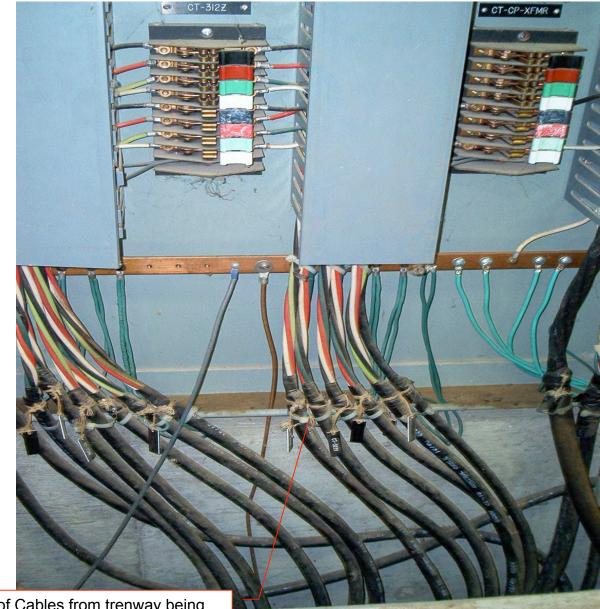
Close-up of Cables from trenway being brought into Control House Junction Box with ground termination details
