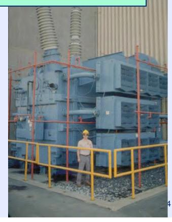
**GIC Caused Transformer Saturation Injects Harmonics**
