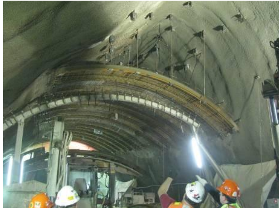
Installing steel forms from Carrier 1
