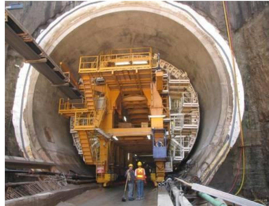
Completed Arch Concrete at the Outlet portal
