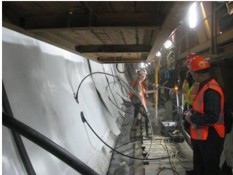
HV testing to verify membrane integrity
