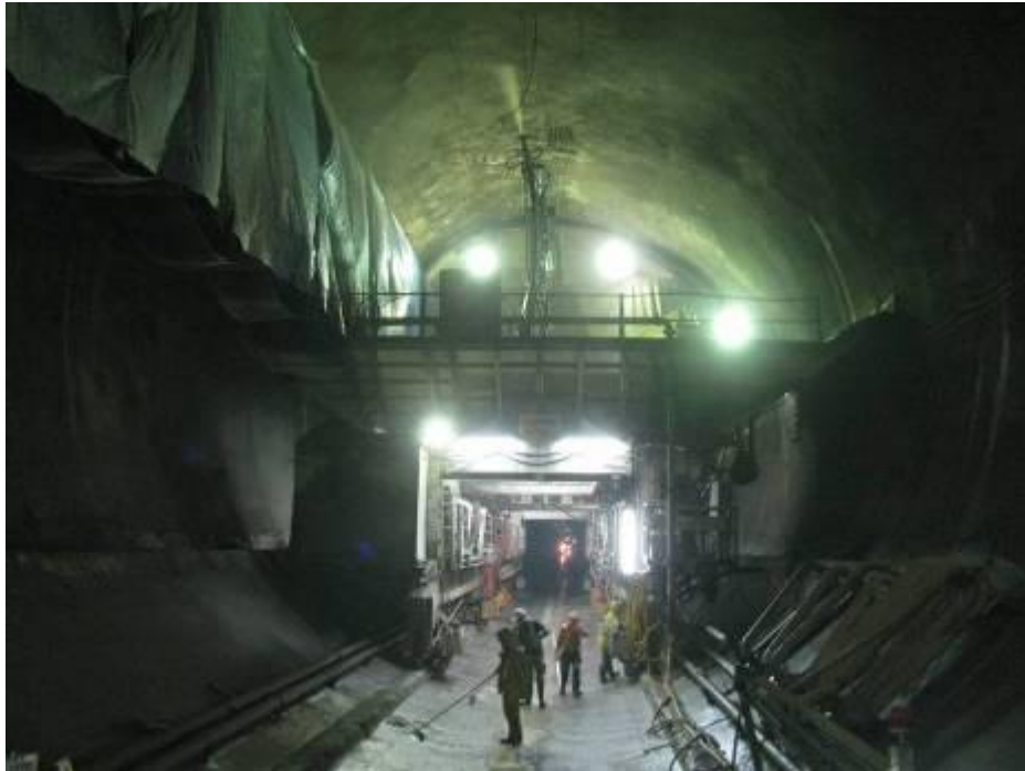
Applying shotcrete from Carrier 2
