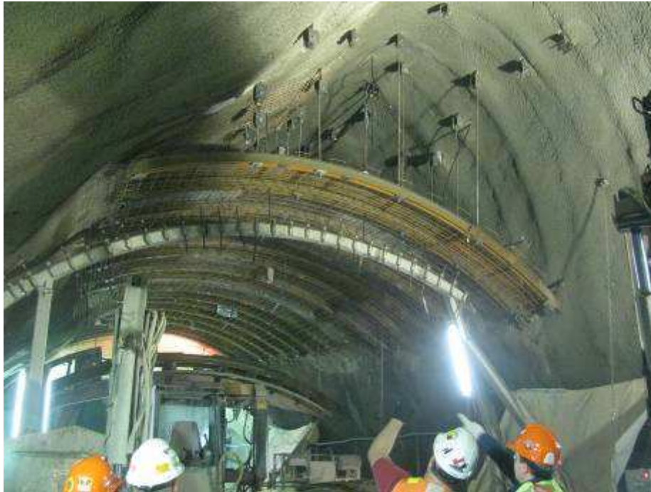
Sacrificial steel forms are suspended in position from rock anchors
