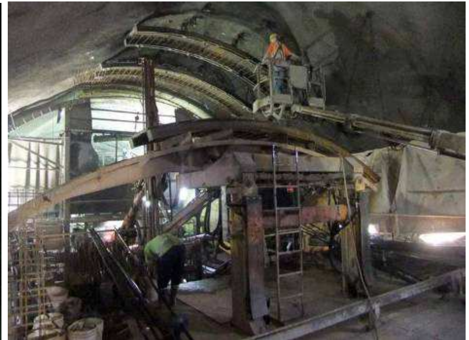
Installing steel forms from Carrier 1
