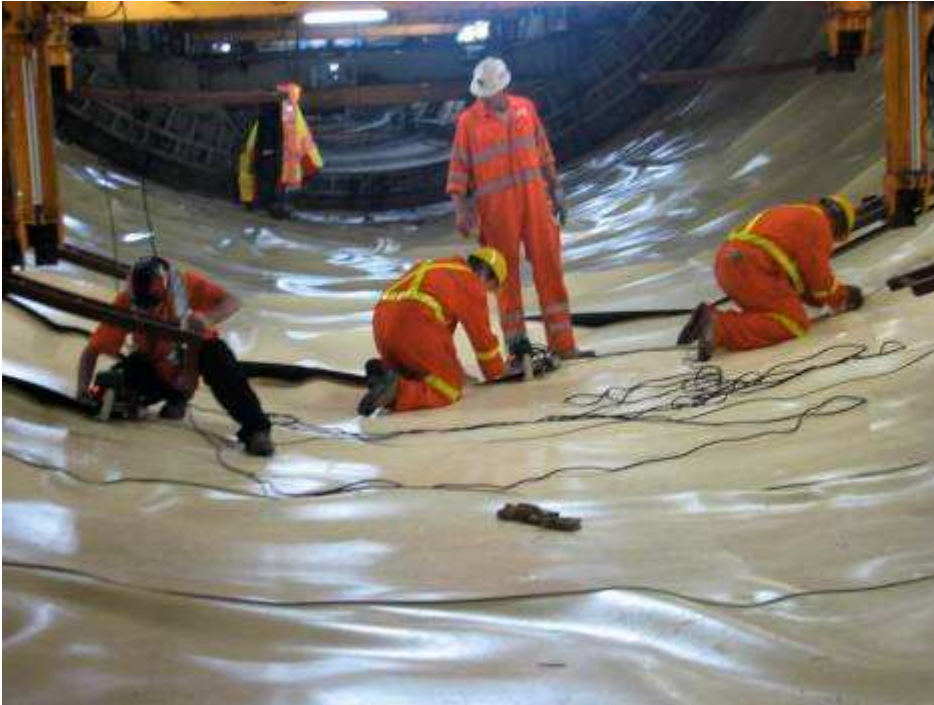
Installing the polyolefin membrane
