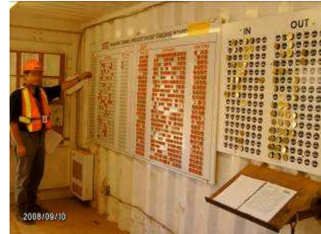
Tag In / Tag Out for Tunnel Access
