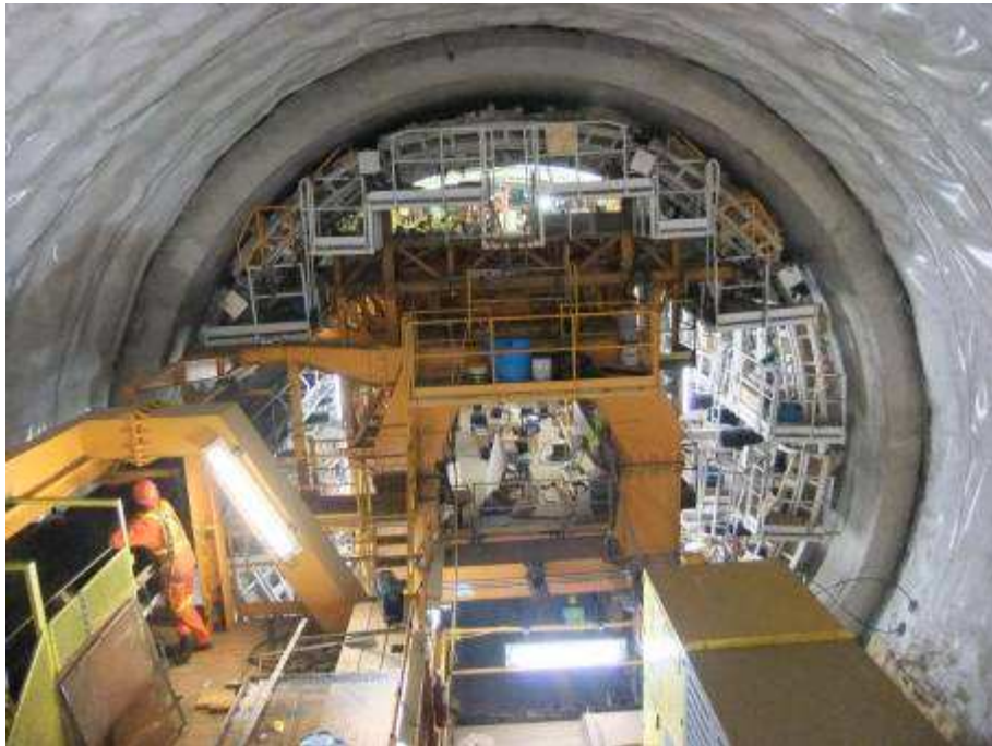
Arch Membrane and Concrete near the Outlet
