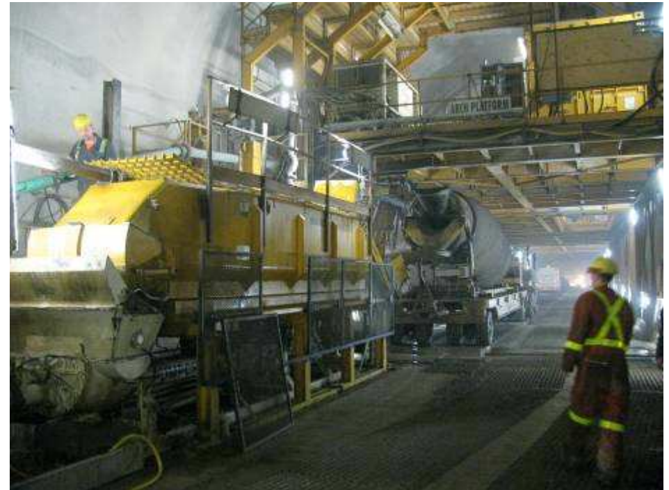
Arch Membrane and Concrete near the Outlet
