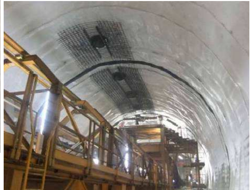
Impermeable membrane installed before the Arch Concrete at the dewatering shafts
