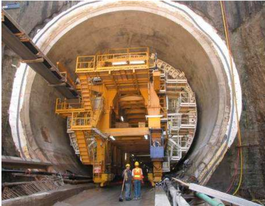
Completed Arch Concrete at the Outlet portal
