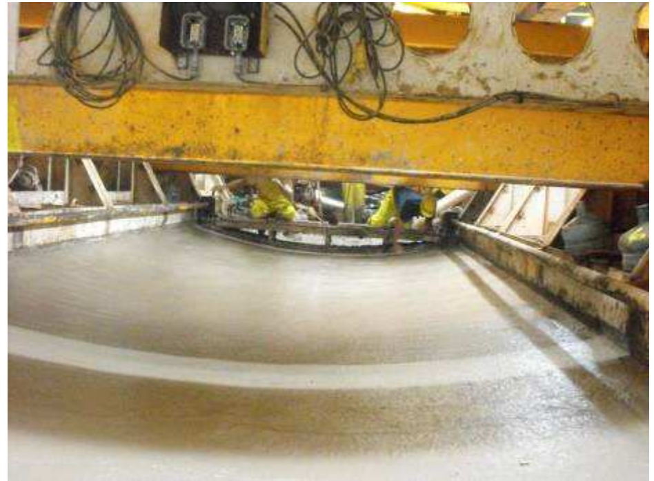
Finishing the invert concrete
