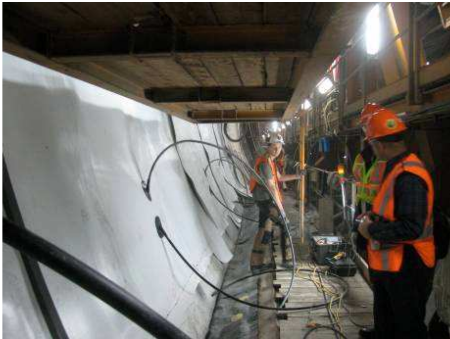
HV testing to verify membrane integrity
