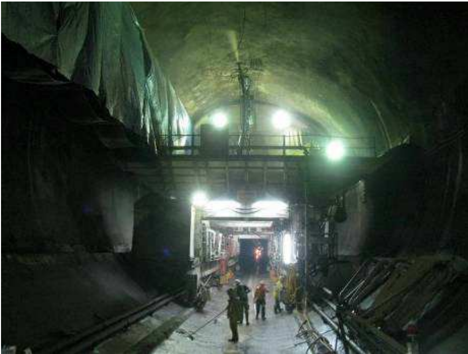
Applying shotcrete from Carrier 2
