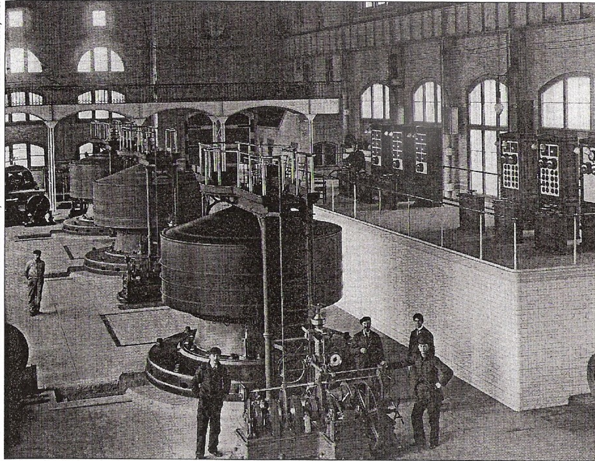
The first three Westinghouse dynamos in Stanford White's "Cathedral of Power" at Niagara Falls in a photo taken April 6, 1896.
