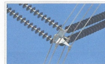
Bundle conductor attachment
