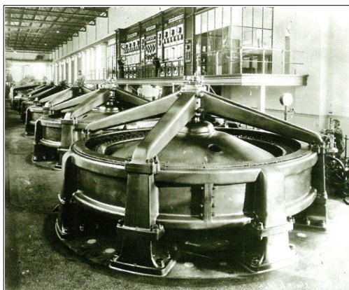
Power house of the Rheinfelden Hydroelectric Power Plant
