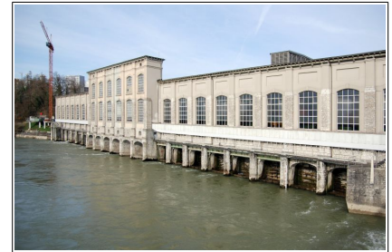
Rheinfelden Powerplant Hydroelectric Power Station
