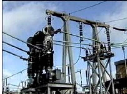
Supplies were affected after the substation fire
