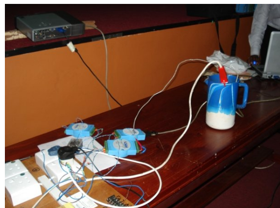
A Programmable Logic Controller Demonstration Circuit
