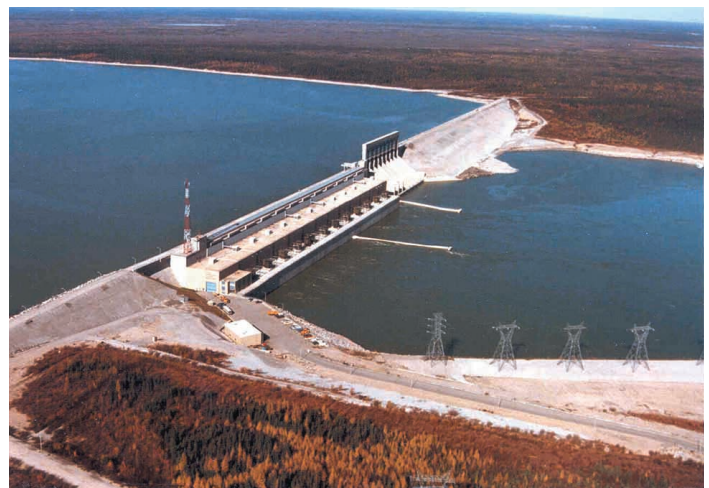
Figure 4: Kettle Plant (Source: Manitoba Hydro)
