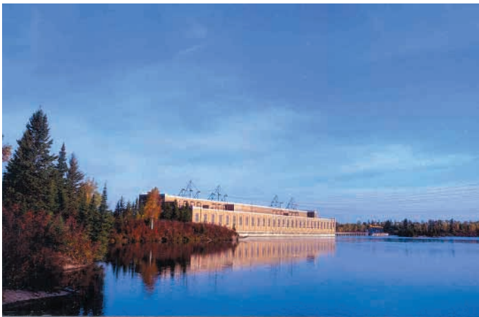
Figure 1: Slave Falls Plant (Source: Manitoba Hydro)
