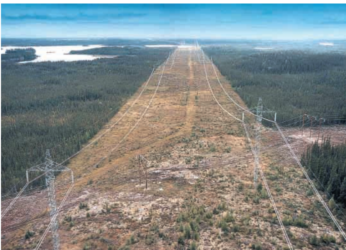
Figure 6: 500 kV HVDC transmission line over the new 230 kV North Central transmission line from Kelsey Generating Station. (Source: Manitoba Hydro).
