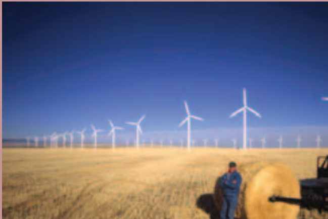
Fig. 4 Summerview wind farm in Pincher Creek (Alberta) Photo Courtesy of TransAlta Wind
