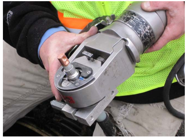
Figure 5: Swaging on injection adaptors during the Sustained Pressure Rejuvenation process.
