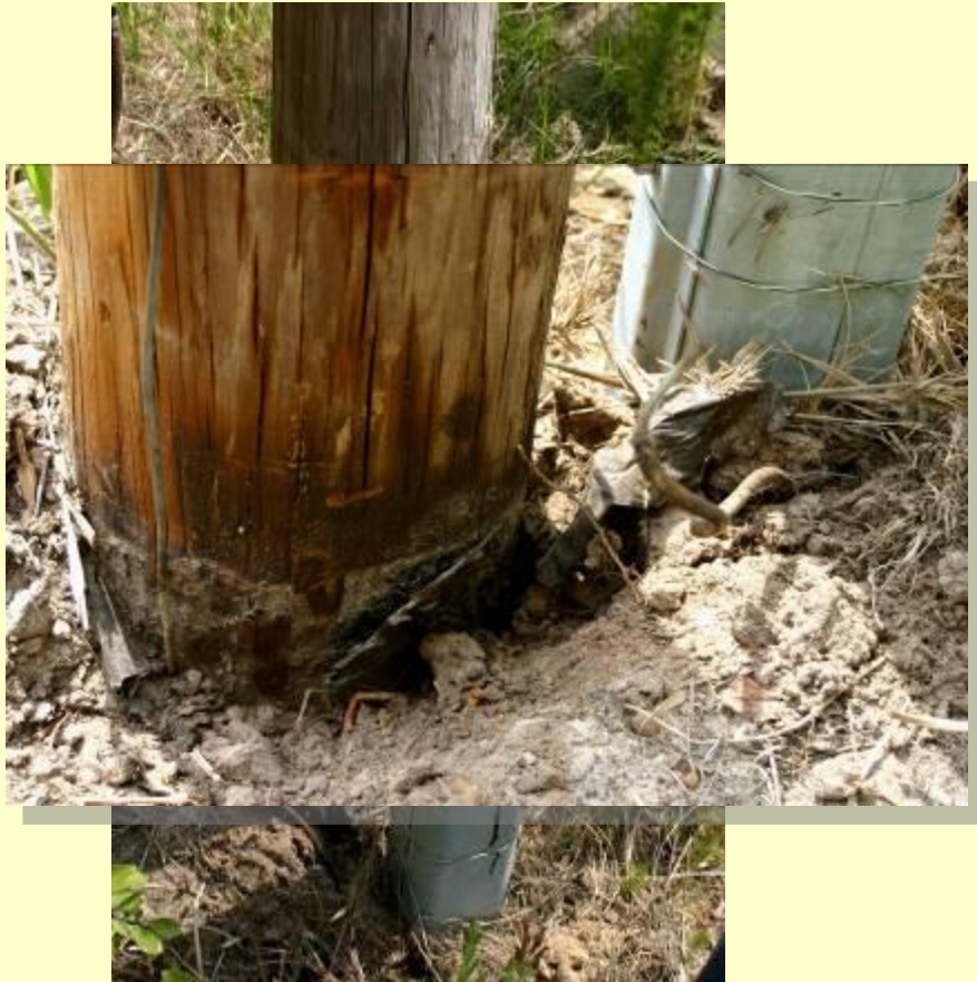
Noisy Telephone Pedestal Faulty Ground – Atlanta, GA
