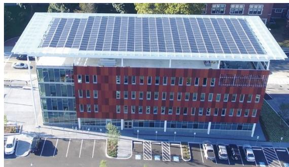
Fig 1. A multistory building with rooftop solar power.
