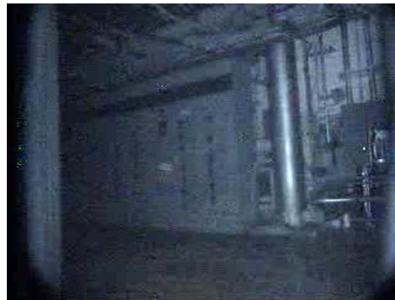
1 st floor of R/B Unit 2
