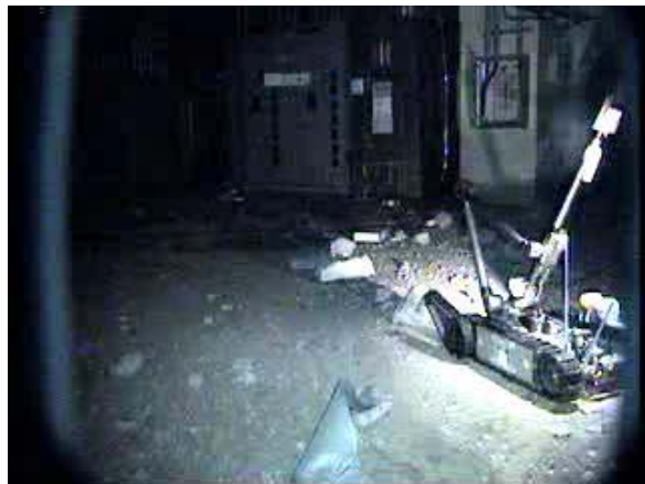
1 st floor of R/B Unit 1
