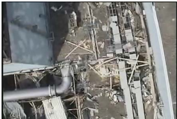
Top View of R/B Unit 1
