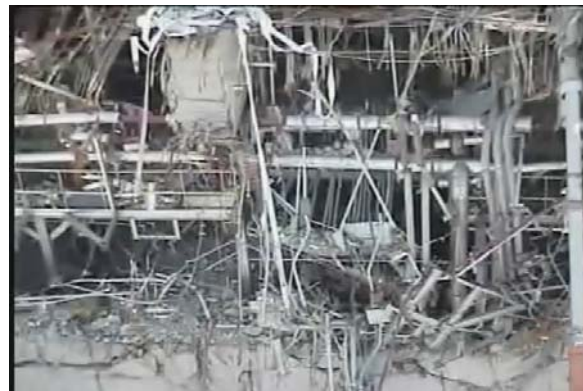
Top View of R/B Unit 3
