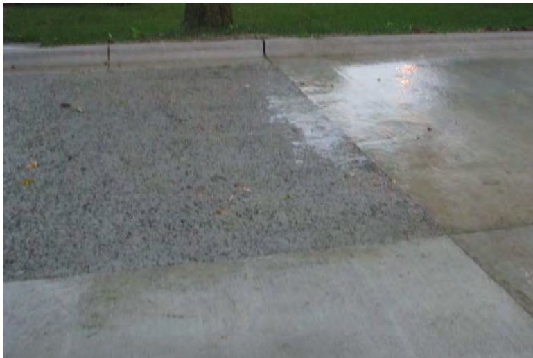
Pervious Pavement for Driveways
