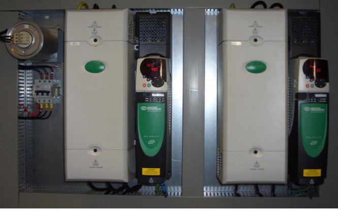
Fig. 2. Rotor circuit back-to-back converter
