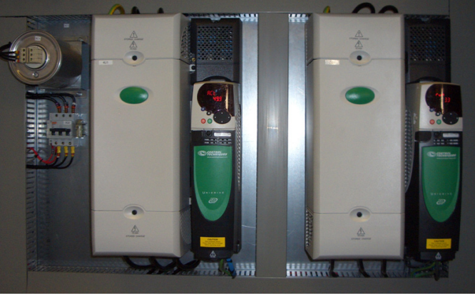
Fig. 2. Rotor circuit back-to-back converter
